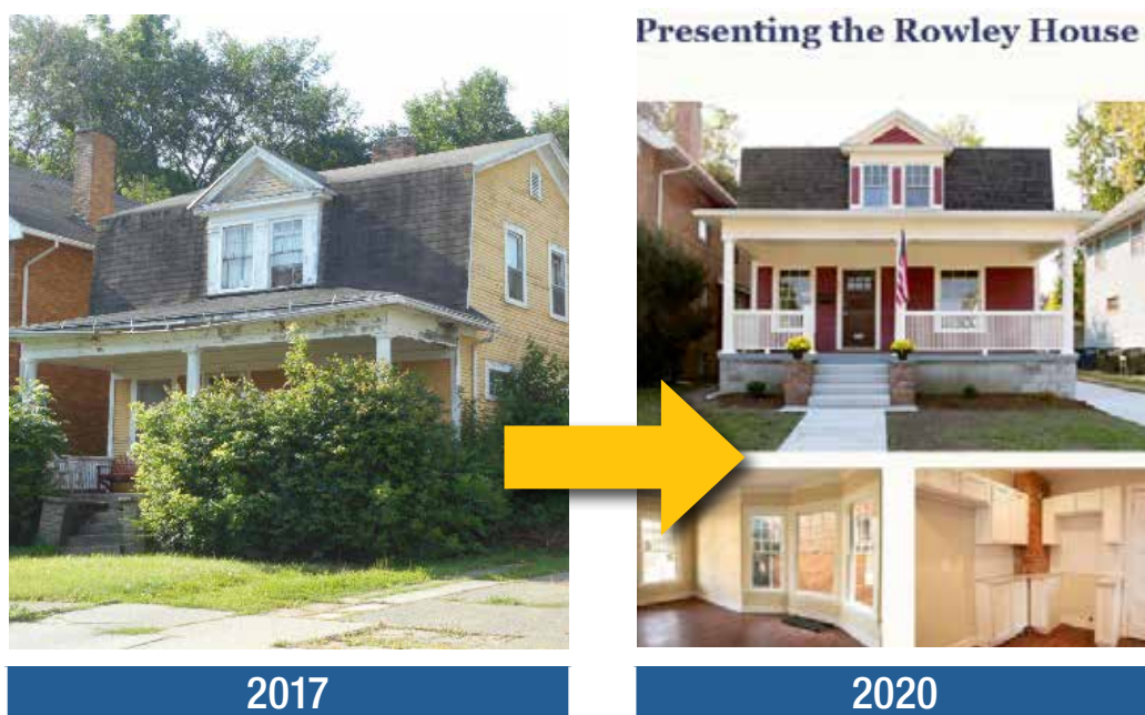
FIGURE 19: The Rowley House Project, Lucas County Land Bank
